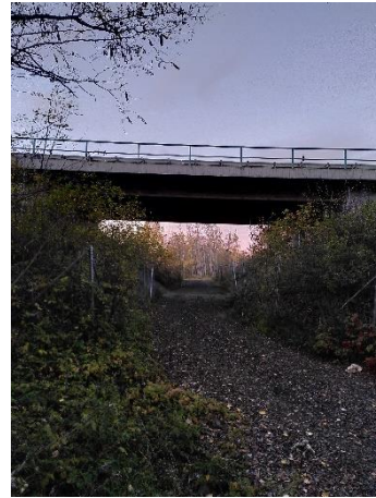
ANNEX 19: UNDERBRIDGE B2 BETWEEN LAKE ZWENKAU AND AIRPORT FOR SPORTS AEROPLANES.
